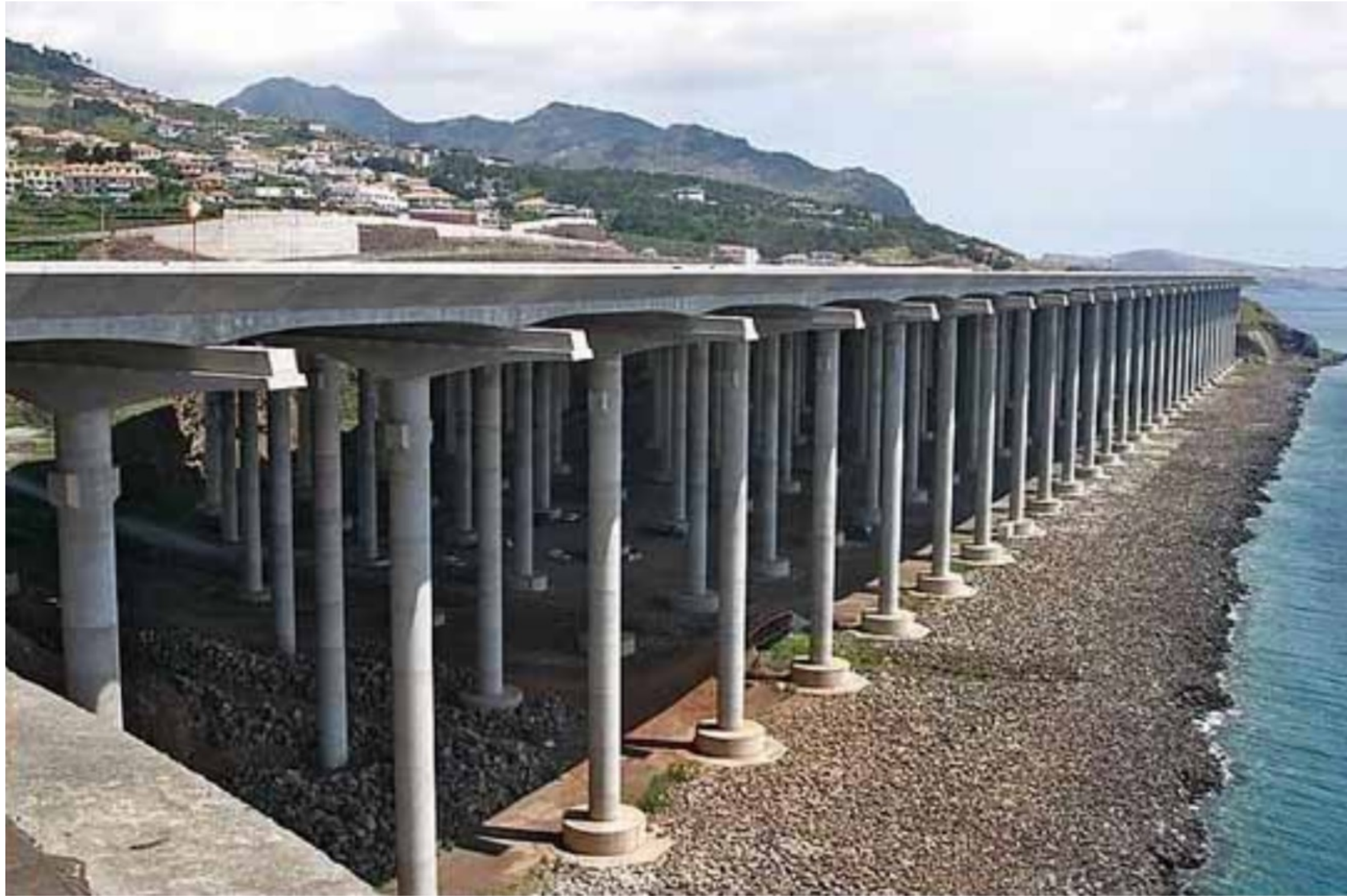
Photo of Runway Bridge at Madeira International Airport in Madeira, Portugal. The Runway Bridge is 3,280-feet long, 590-feet wide with 180 pillars each approximately 187-feet tall.
